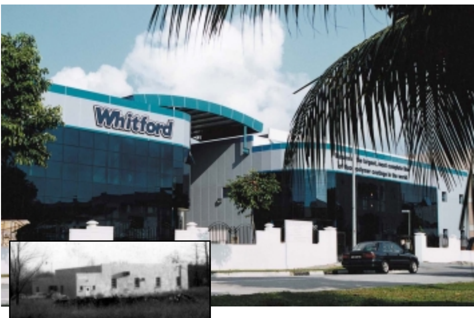
New Singapore Plant and Original Whitford Building (inset)
